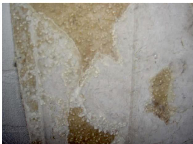
This is a polyester resin backed tile which was installed in an external application with a cement based adhesive. Over a two year period the resin was decomposed by the cement in the adhesive resulting in breakdown and de-bonding.
