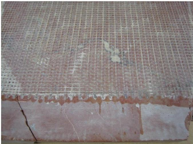
This example shows double layer of reinforcing mesh and tile still cracked.
