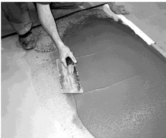
The mixed material is spread and trowelled into shape to provide falls or form a ramp.
