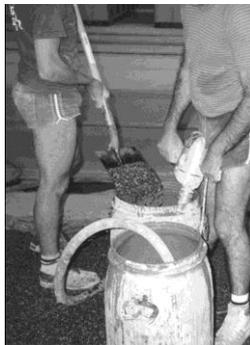
Mixing is performed with a high speed mixer such as a drill fitted with an ARDEX mixing paddle. Normal mixing is done for 2 minutes, and then the aggregate/sand is added and mixing continued till the aggregate is wet out.
